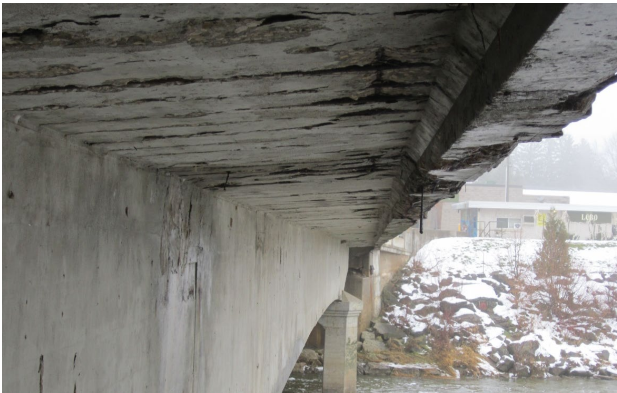
View of deterioration present on sidewalk soffit along the east limit of the bridge
