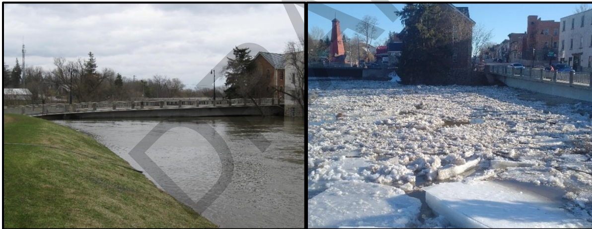
Figure 4.2 Teeswater River Bridge Flooding and Ice Jams
