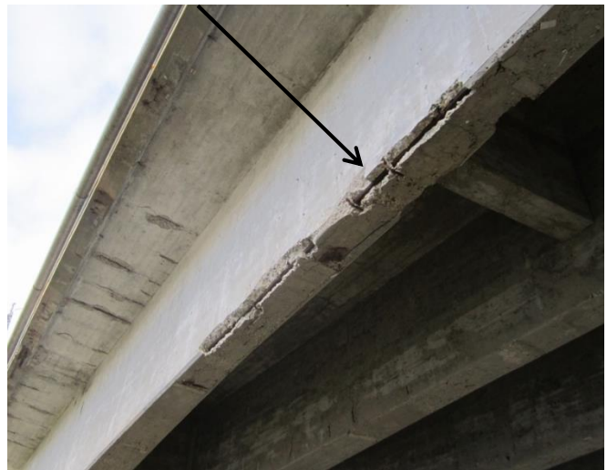
BEAM DETERIORATION
